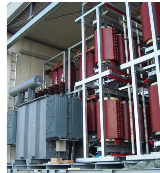
**PSM Transformer Arrangement** | The PSM transformer provides the AC power to each PSM module in the switching module assembly of the HVPS units.
