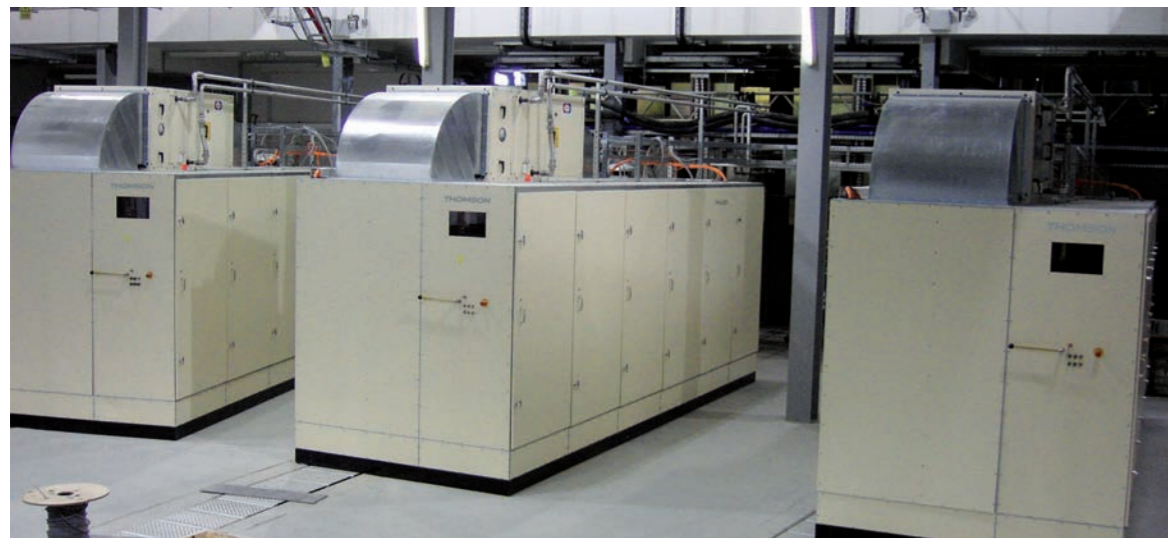
Ampegon systems during installation at DLS.
